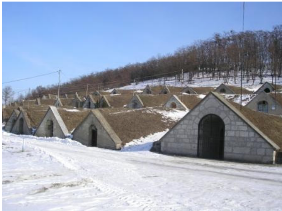
The Gombos-hegyi cellar row in Herceghút
