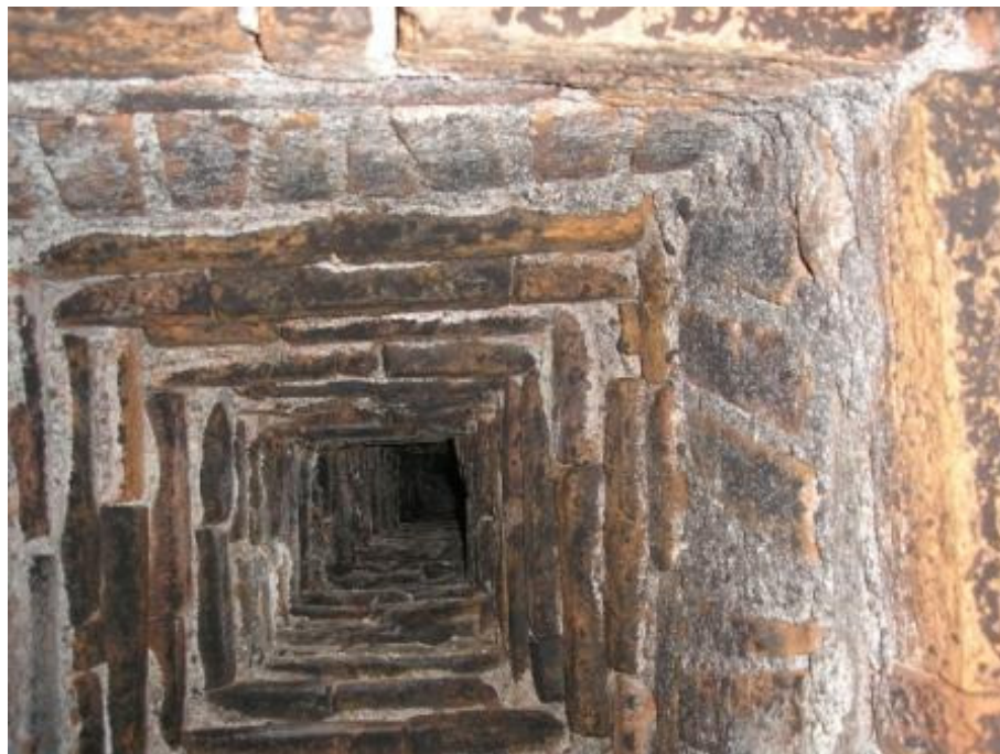
Brick-faced air shaft in Sátoraljaújhely
