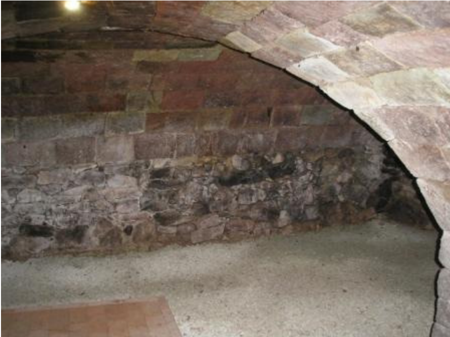
Arch in Mád; strengthened later
