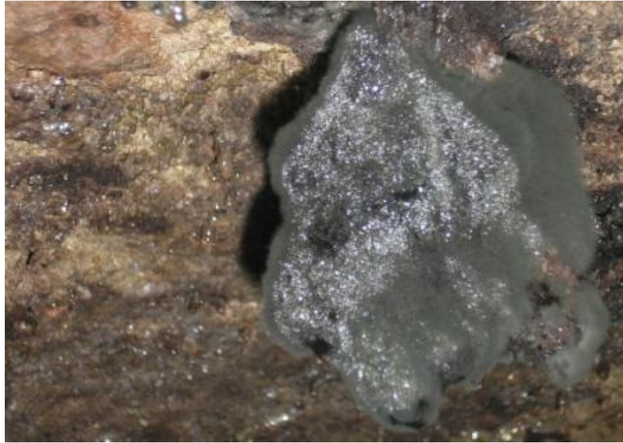
Condensation of humidity on the cellar mould
