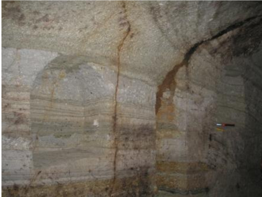
A recently excavated cellar in Herceghút
