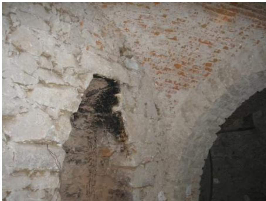
Stone and brick together near the entrance to a cellar in Bodrogkeresztúr
