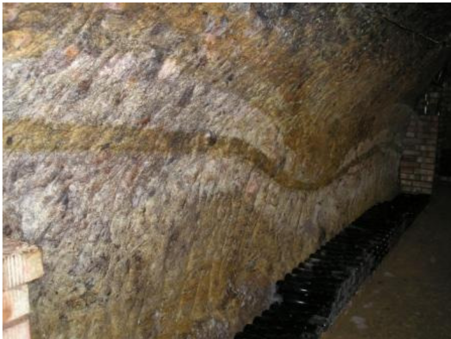
These layers became visible after widening of this cellar in Tállya
