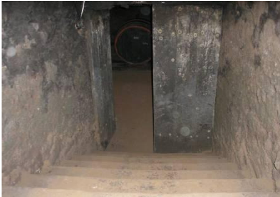
Doors used for air regulation
