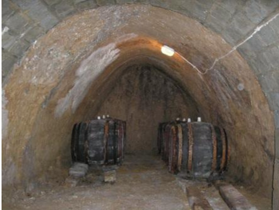
The original Gothic semicircular arch in Erdőbénye (recently strengthened)
